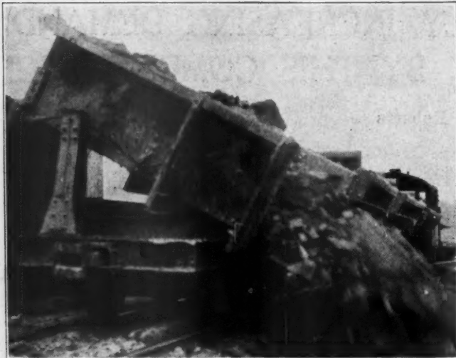
Discharging to Crusher
